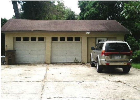
3. View of existing garage, looking E
