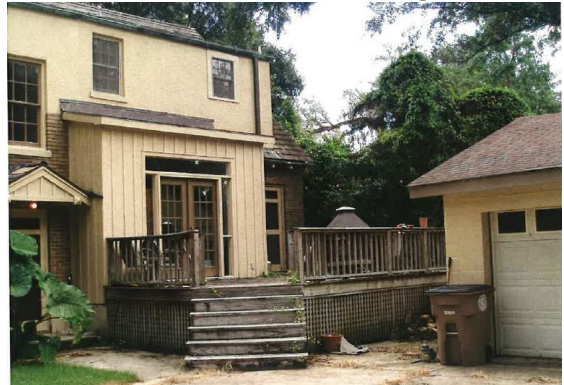
4. View of rear elevation and garage, looking NE
