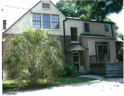
2. View of south (rear) elevation, looking NE
