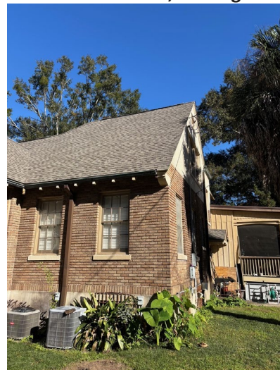
6. View of west and south elevations, looking NE
