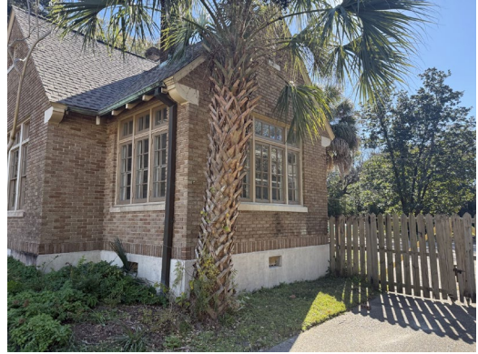
2. View of west elevation, looking SE
