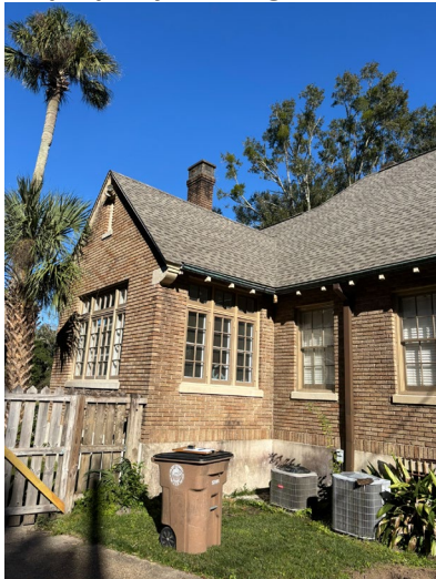
3. View of west elevation, looking NE
