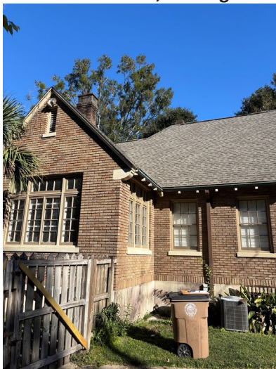
5. View of west elevation, looking E
