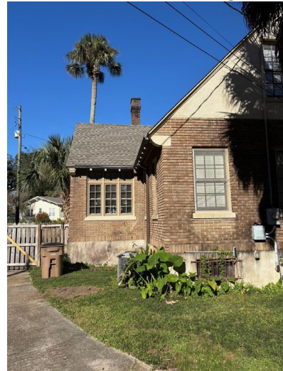
4. View of south elevation, looking N
