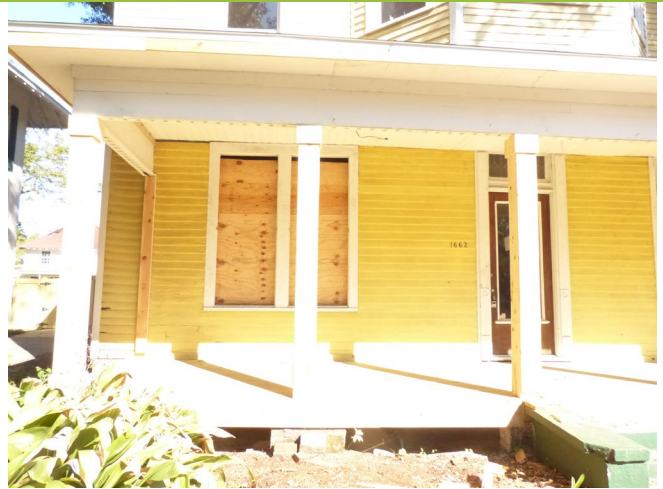
2. View south to west end of front porch
