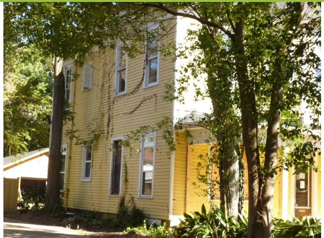
8. View northeast to west elevation
