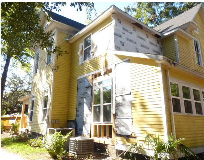
5. View southwest to east (left) and north (right) elevations
