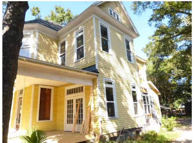
4. View northwest to south (left) and east (right) elevations
