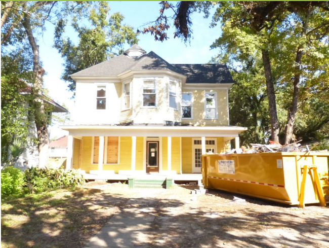
1. South elevation (façade)
