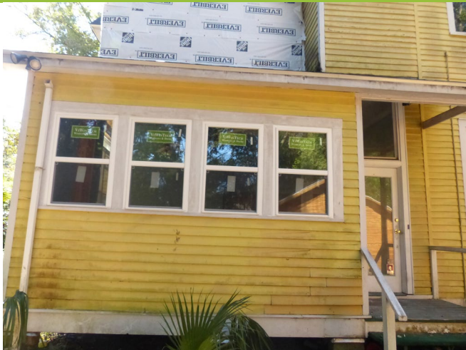
7. Detail: replacement windows on enclosed rear porch
