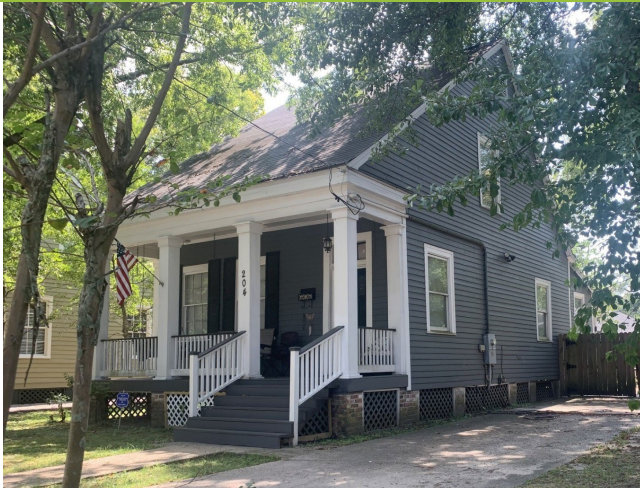
1. View of property looking southwest
