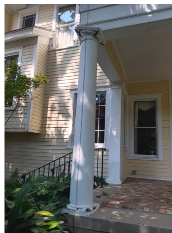
4. Details of column on southeast end of porch.
