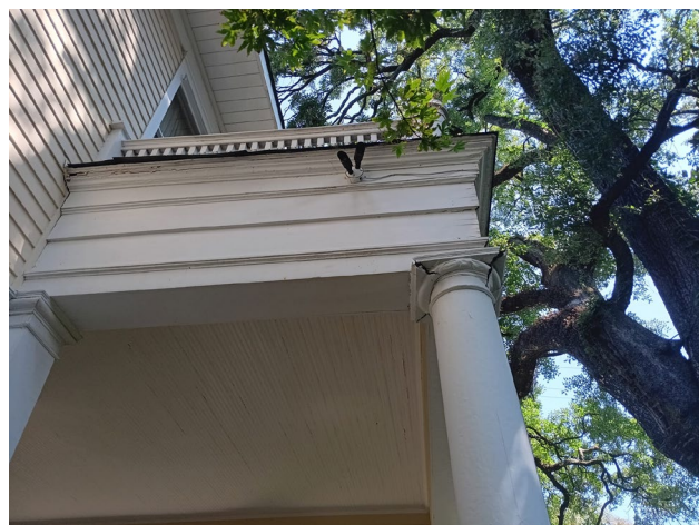
5. Detail of column cap on southeast end of porch.
