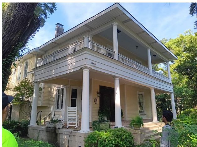
3. View of porch looking southwest.
