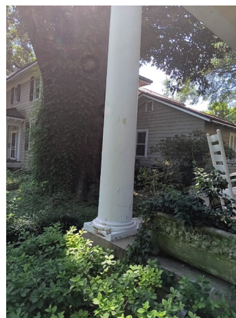
6. Detail of column on northeast end of porch.
