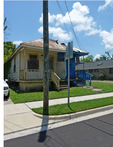
2. View of property, looking southwest
