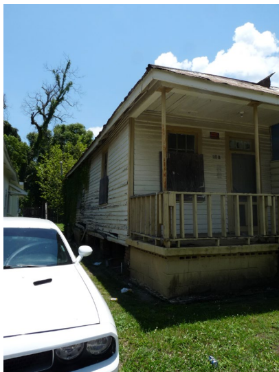
5. View of façade and east elevation, looking southwest.
