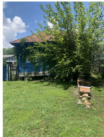
6. View of rear elevation, looking north.
