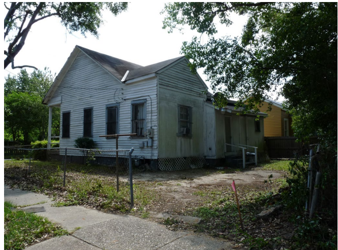
6. View of proposed parking area, looking southwest
