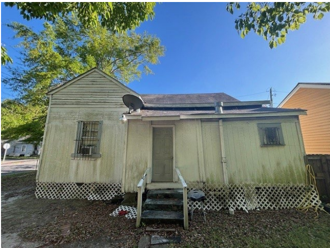
5. View of rear elevation, looking south
