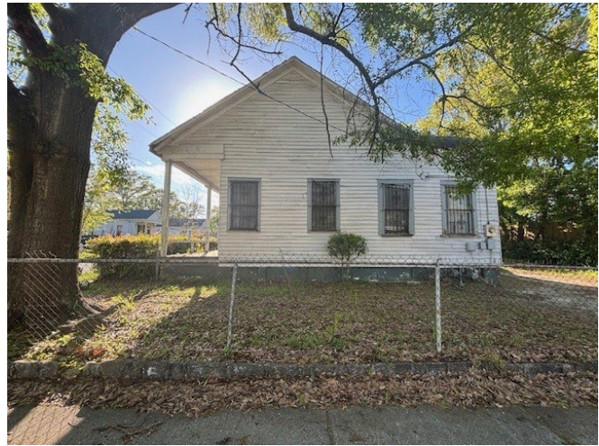
4. View of east elevation, looking west
