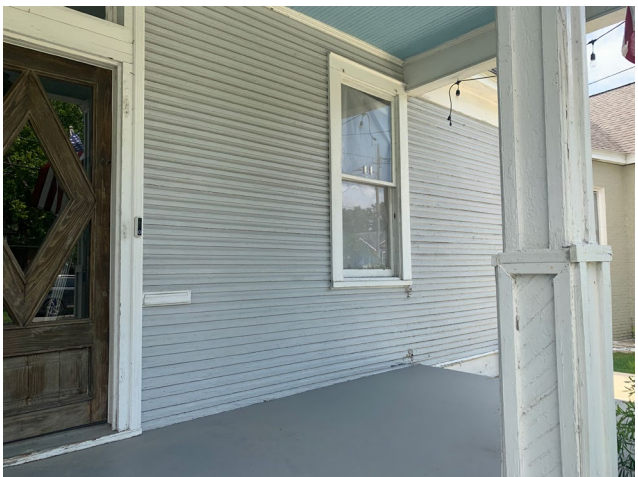
6. View of façade siding
