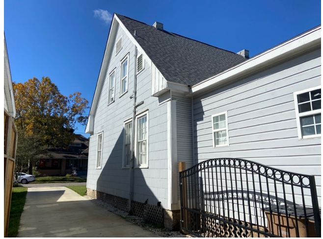
2. View of south elevation, looking northwest. Note asbestos siding on original block and fiber cement on one-story rear addition.
