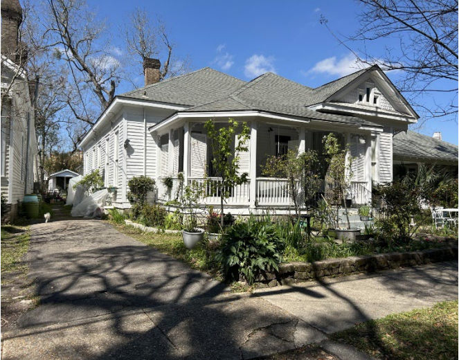
1. View of property, looking NW.
