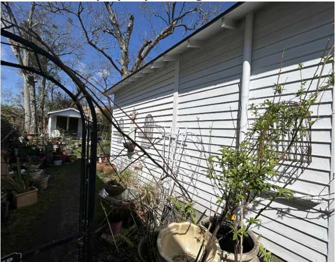
3. View of west end of south elevation with addition, looking NW.
