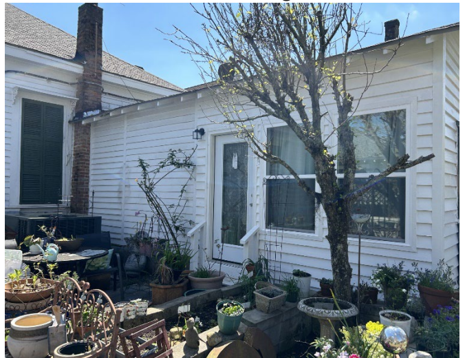
6. View of north elevation, looking SE.
