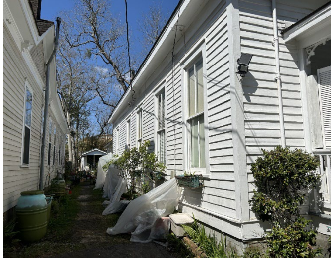
2. View of south elevation, looking NW.
