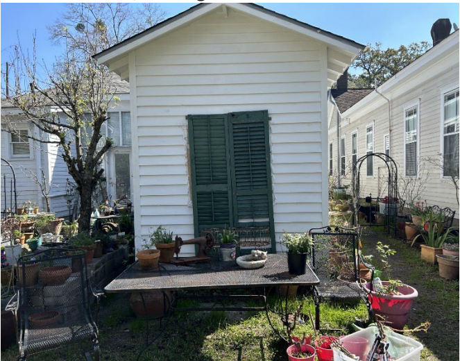
5. View of west elevation, looking E.
