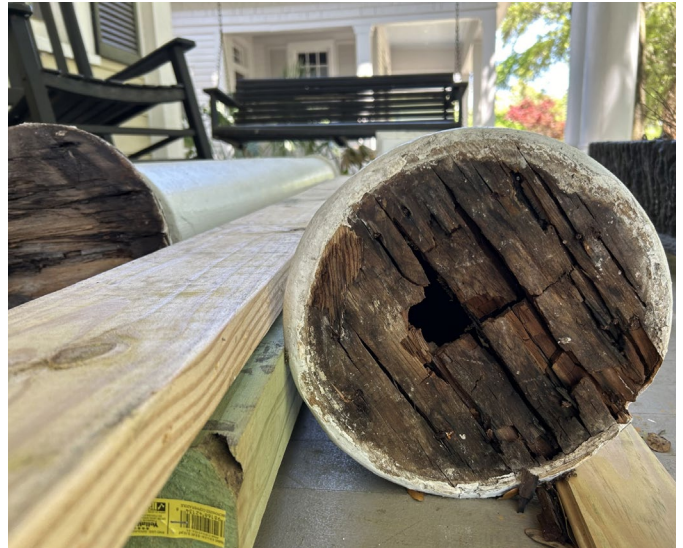
4. Detail of deteriorated column 1
