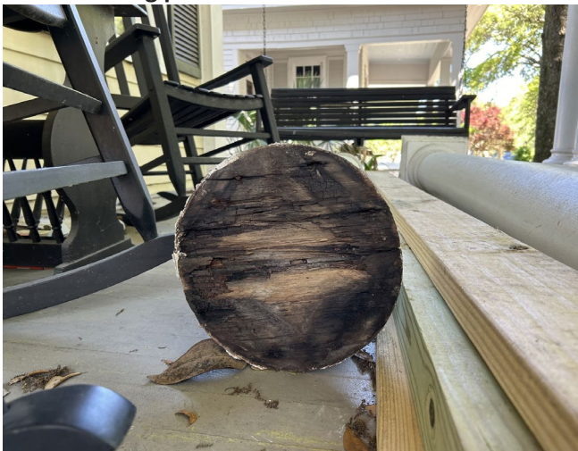
5. Detail of deteriorated column 2
