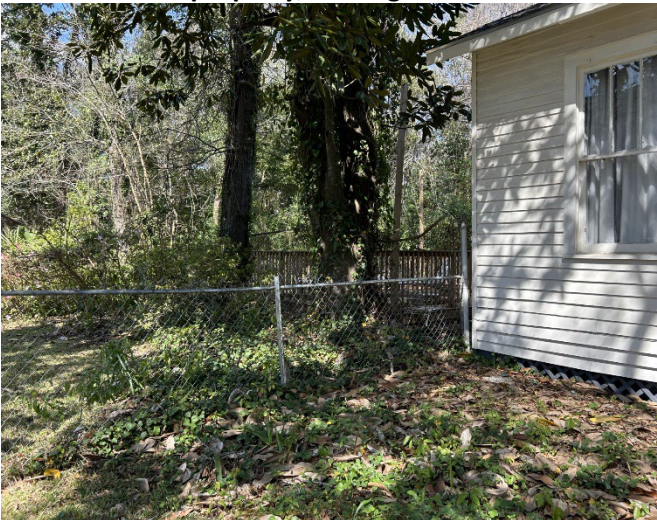
3. View of rear of lot, looking NW.
