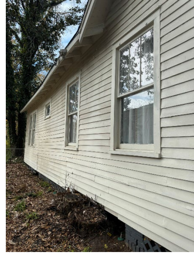
2. View of south elevation, looking NW.
