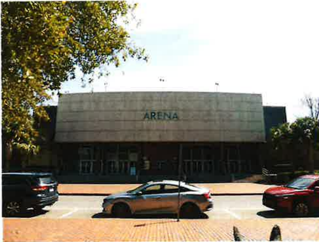
7. View south to north elevation (façade) of Civic Center arena/auditorium from Malaga Square
