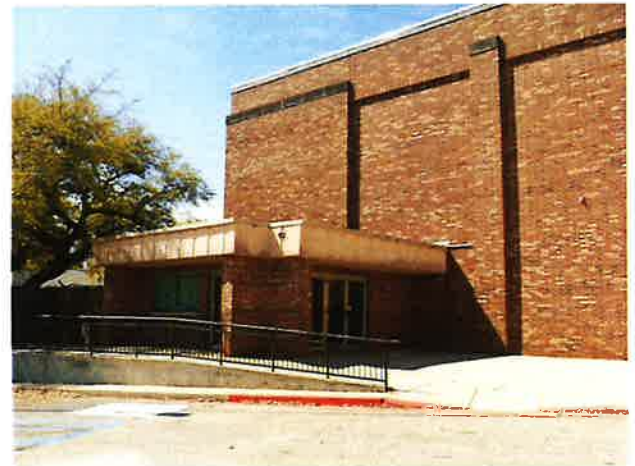
24. View northwest to c. 1990 addition to south (rear) elevation of Civic Center expo hall
