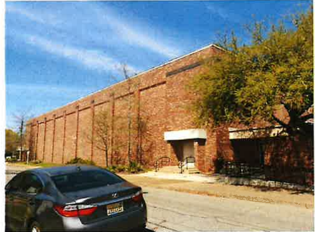
22. View north-northeast to west elevation of Civic Center expo hall
