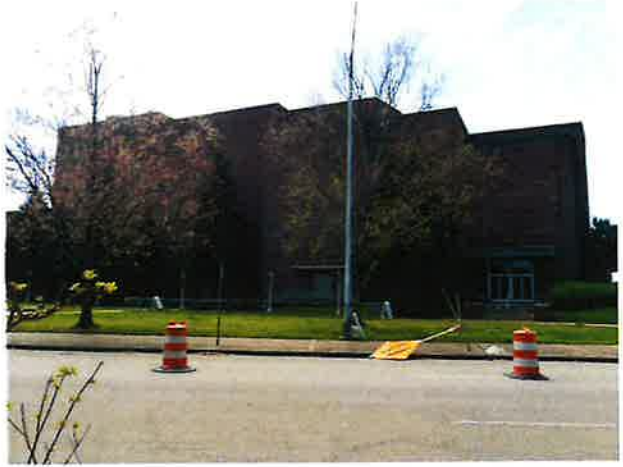
2. View west to the east elevation of the Civic Center theater
