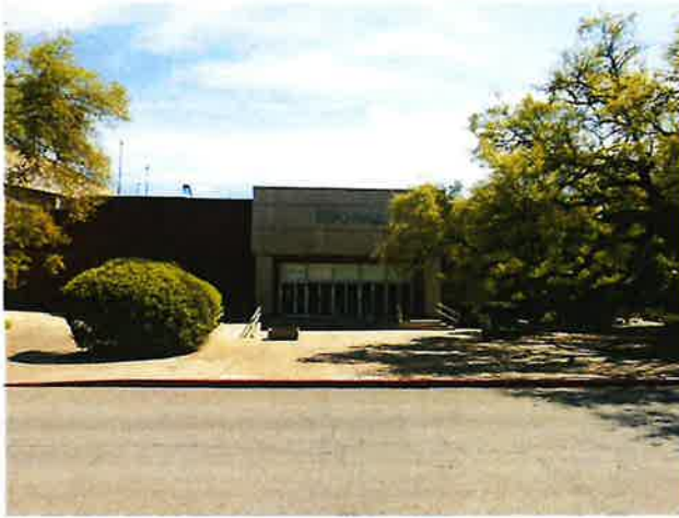
19. View south to north elevation (façade) of Civic Center expo hall
