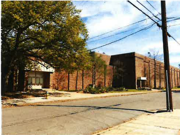
21. View southeast to west elevation of Civic Center expo hall
