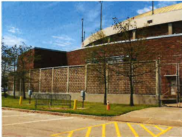
15. Detail: breeze block enclosure on south side of Civic Center arena/auditorium
