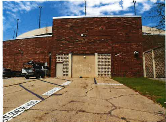
16. partially enclosed vehicle opening on south side of Civic Center arena/auditorium
