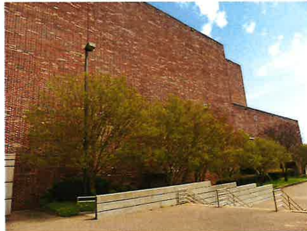
5. View southeast to west elevation of Civic Center theater
