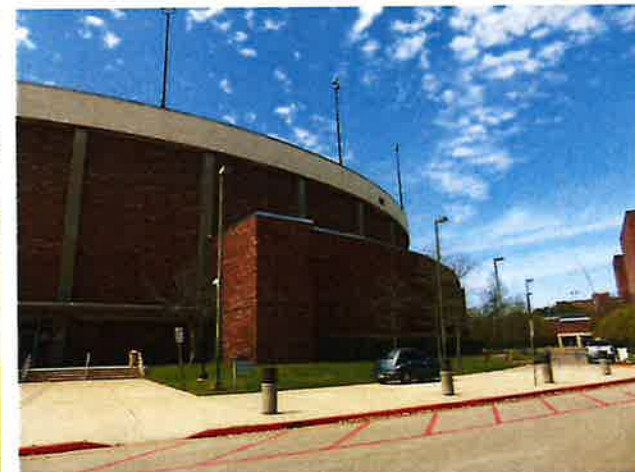
12. view north to southeast side of Civic Center arena/auditorium; theater at right
