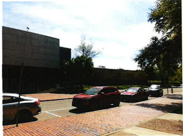
8. View southwest to concourse between Civic Center arena/auditorium and expo hall
