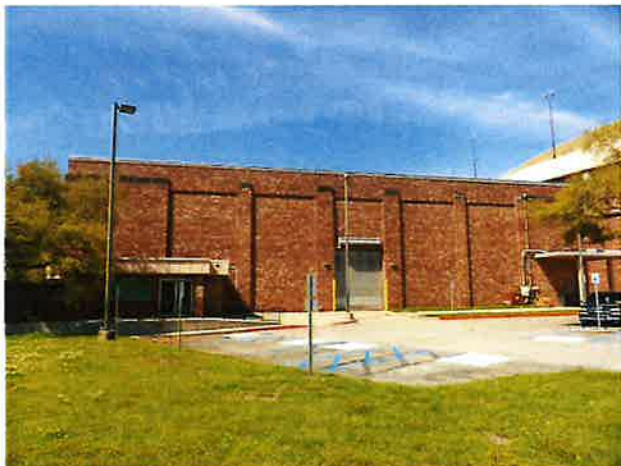
23. View north to south (rear) elevation of Civic Center expo hall
