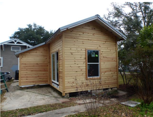
5. View of west elevation of addition
