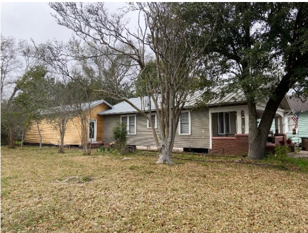
3. South elevation, post alterations
