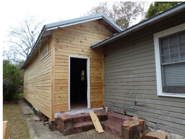
4. East and south elevations of addition
