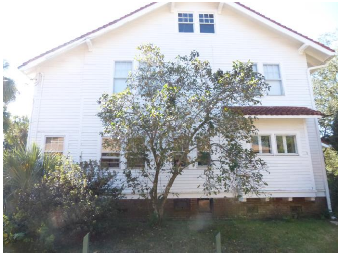
4. North elevation; subject windows at 1 st floor center
