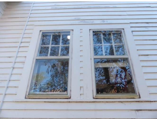
5. Detail: westernmost pair of windows proposed for replacement
