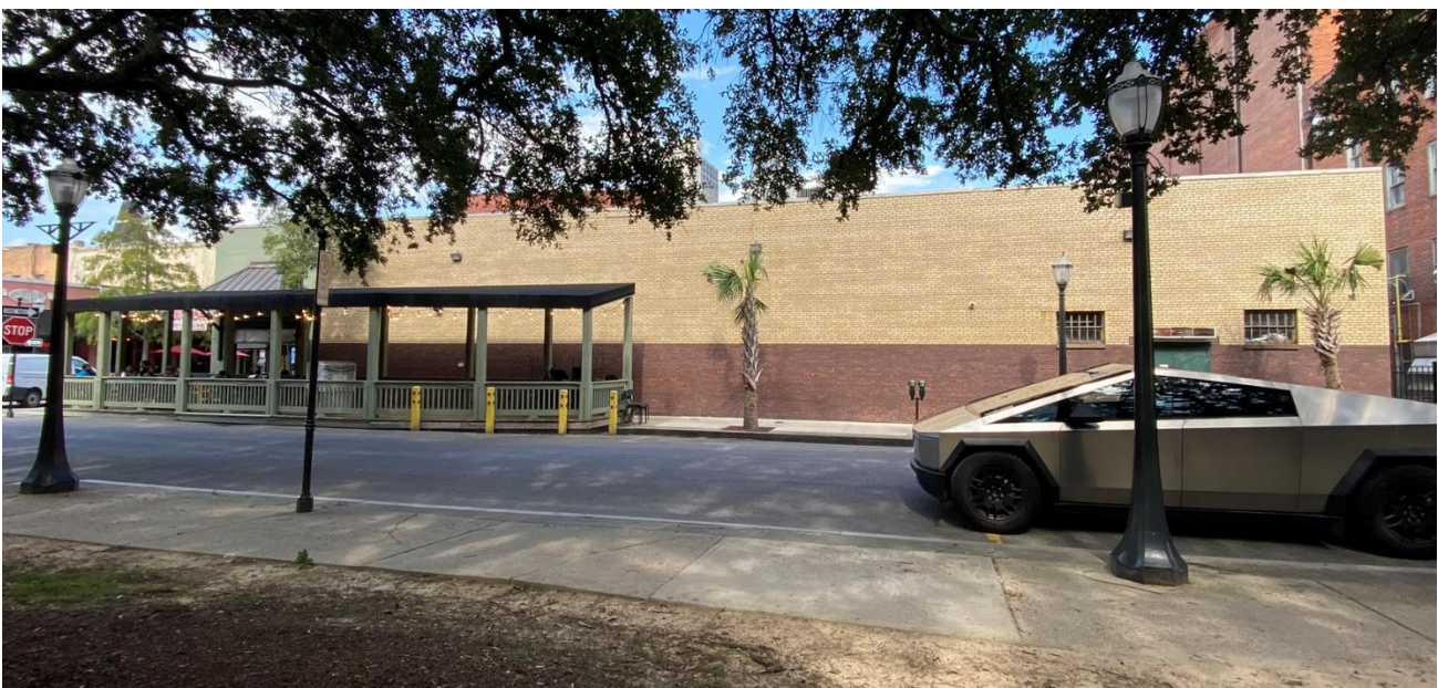
5. West elevation, looking east
