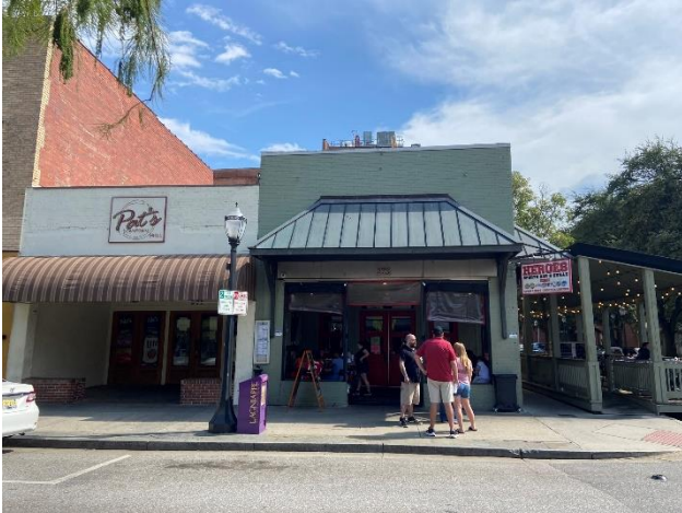
1. North (primary) façade, looking south
