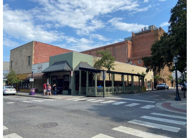
2. North and west elevations, looking southeast
