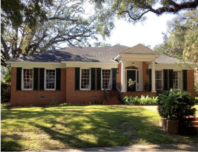
1. Primary façade, looking southwest
