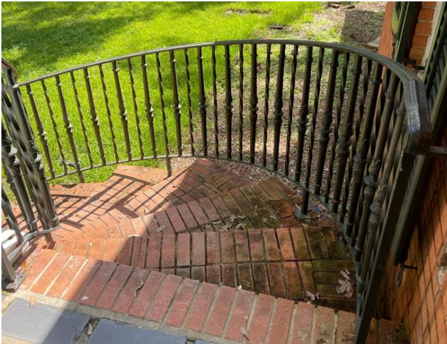
3. Detail of east stair, looking southeast
