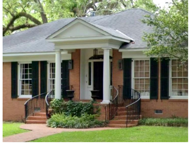
2. View of entry porch and existing stairs, looking south
