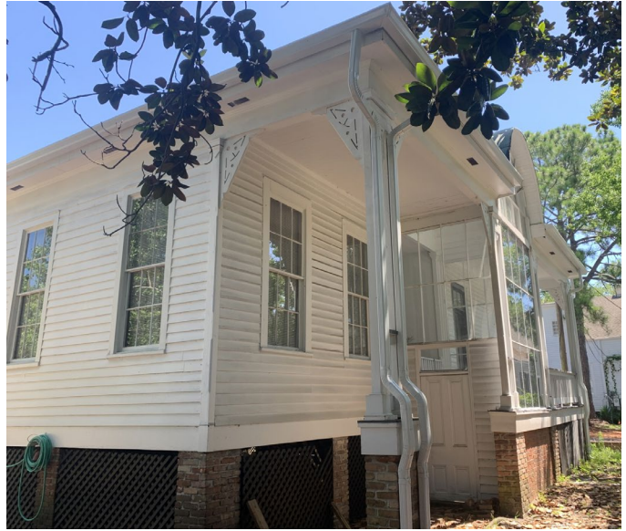
2. Southwest corner, showing location of porch reconstruction. Note window to be replaced with door and lower door and transom to be cut down.
