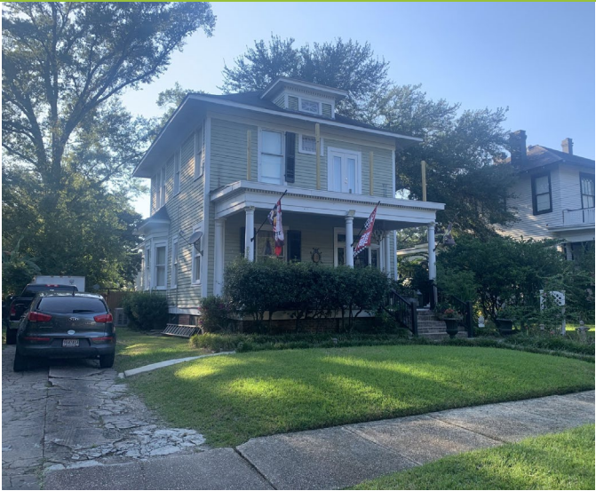
1. View of property, looking NW
