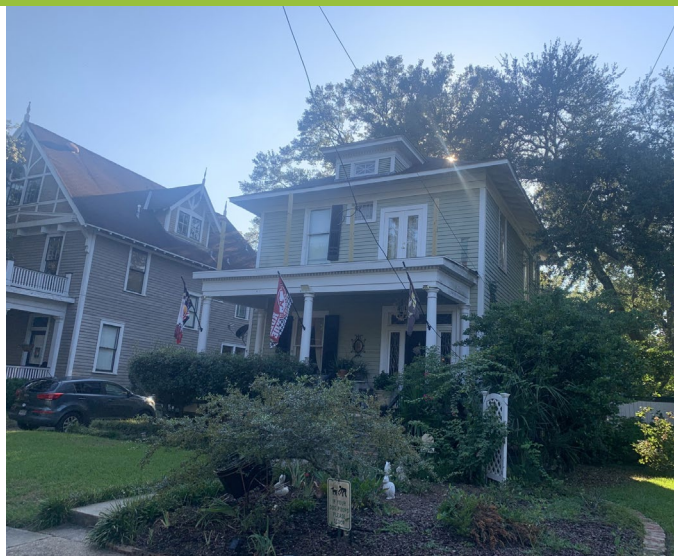
2. View of property, looking SW
