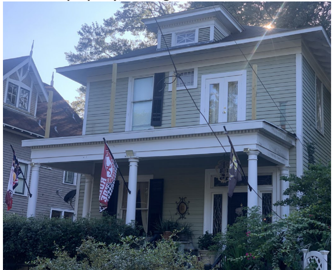
4. View of work on second-story façade, looking SW
