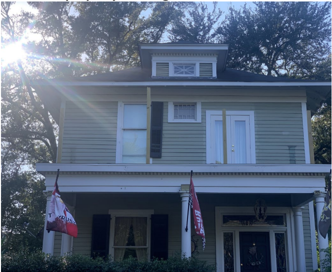
3. Detail of work on second-story façade, looking W
