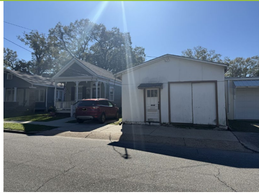
2. View of property, looking S
