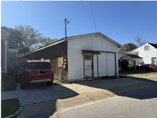
3. View of ancillary structure, looking SW
