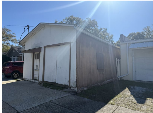
4. View of ancillary structure, looking SE
