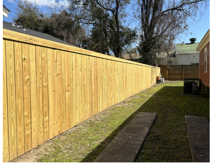
2. View of fence along south property line, looking NE (from neighboring property)
