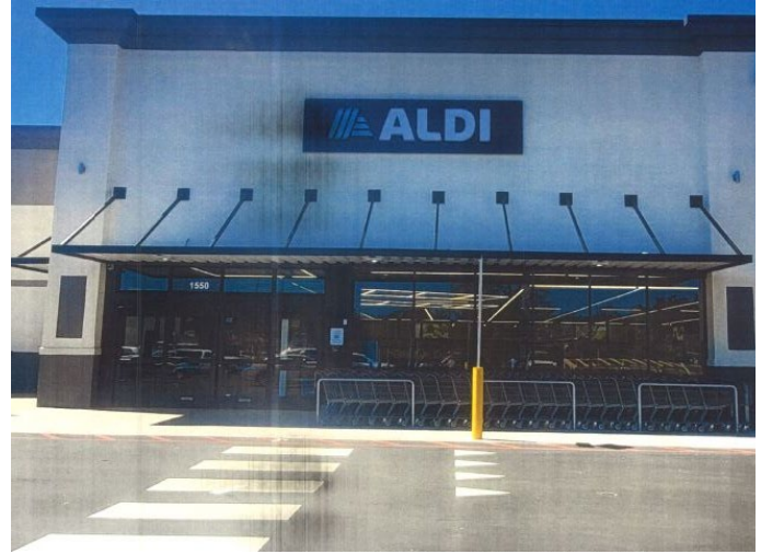
2. View of existing signage on grocery store building façade. Looking west.
