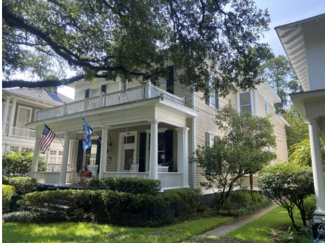
1. View of façade and west elevation, looking SE
