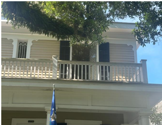
5. Detail of second story original window, submitted by applicant
