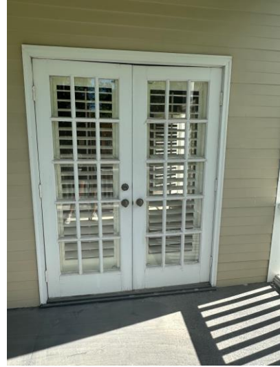
8. Detail of second-story non-historic French doors on rear elevation of addition, submitted by applicant
