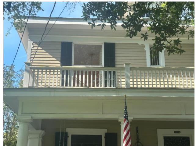
4. Detail of second story original window, submitted by applicant
