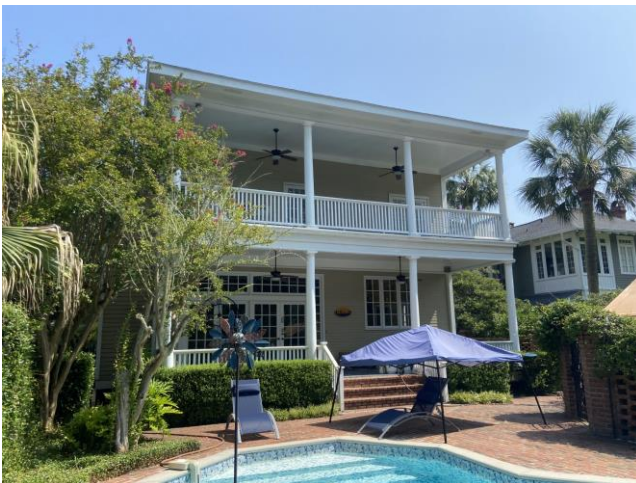
3. View of south (rear) elevation, looking N
