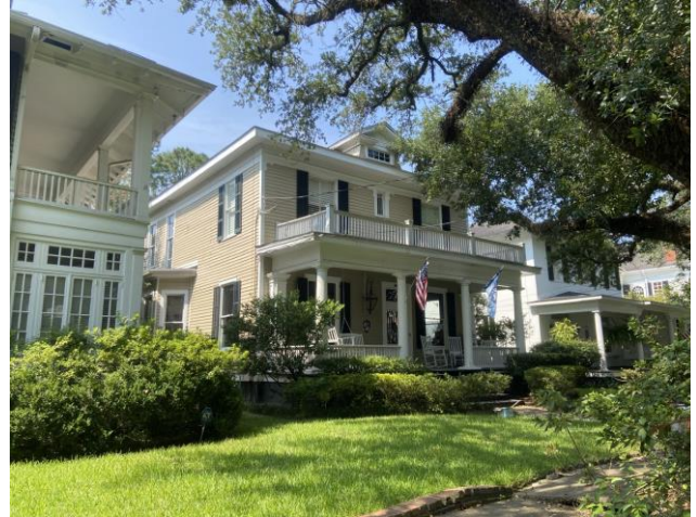
2. View of façade and east elevation, looking SW
