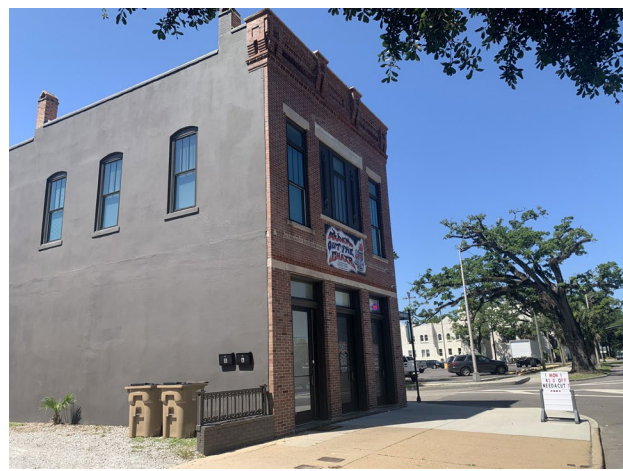
4. 809 Government, adjacent commercial building north of subject lots.
