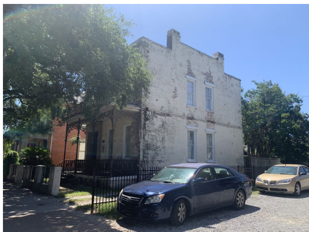
5. 803 Government, adjacent residence northeast of subject lots.
