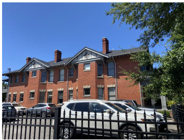
6. 805 Government, adjacent residence northeast of subject lots.
