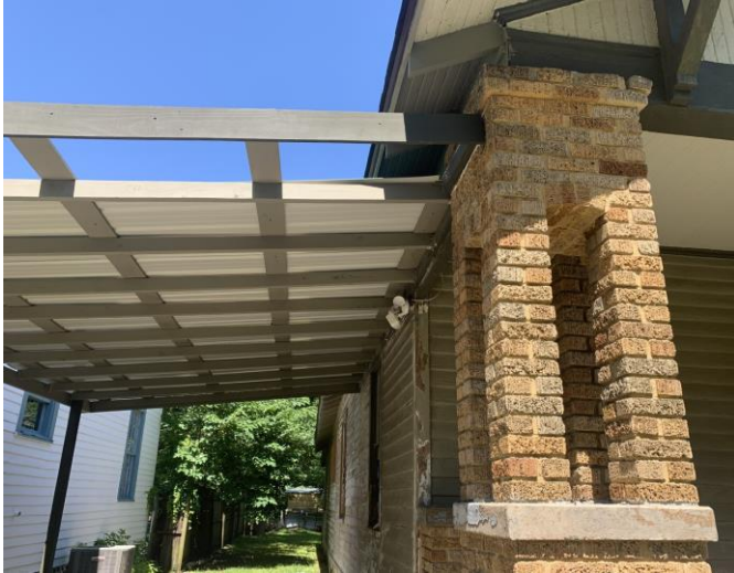
3. Detail of existing/repaired portion of carport.
