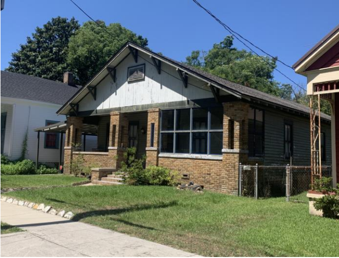
1. View of east façade, looking southwest.
