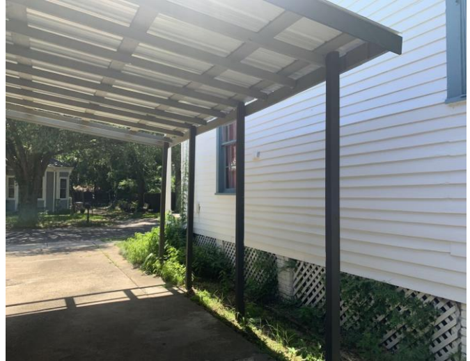
4. View of carport, looking east.
