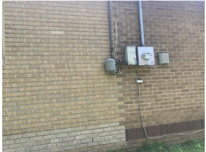
4. Detail: differing bricks on original (right) and addition (left)
