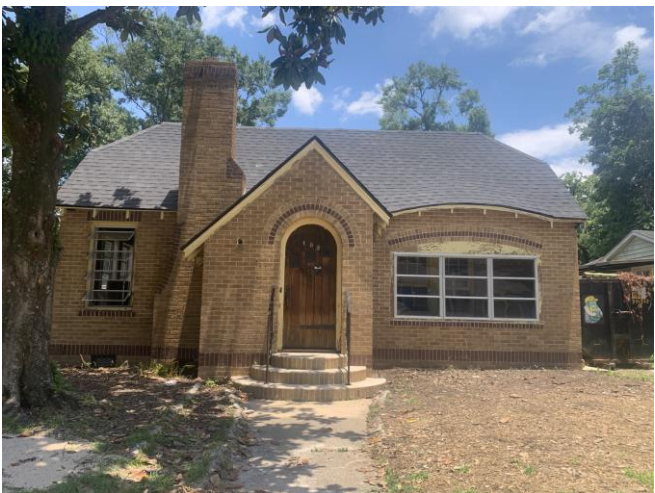
5. Façade view. Note decorative brickwork above entry and at right
