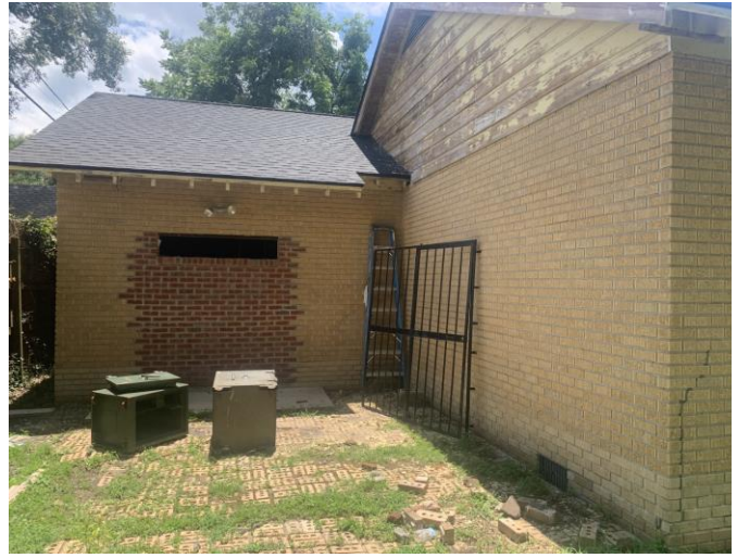
8. View of rear elevation (later addition).
