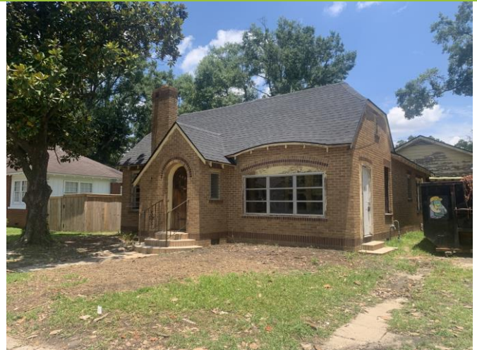
2. View of west façade and south elevation
