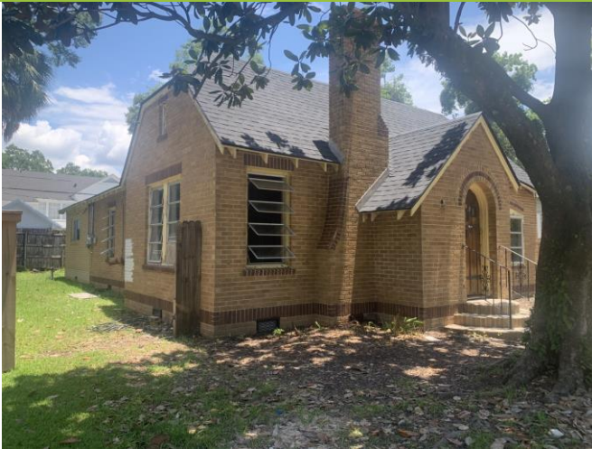
1. View of west façade and north elevation
