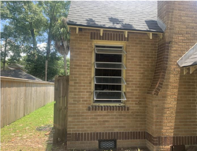
7. Detail of existing replacement window and decorative brickwork.
