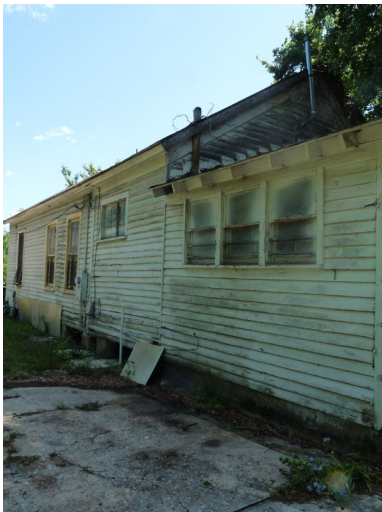
3. View of west elevation, looking NE
