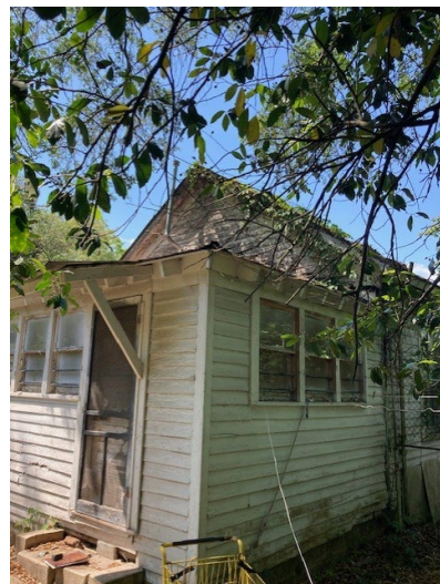
6. View of south and east elevations, looking NW.
