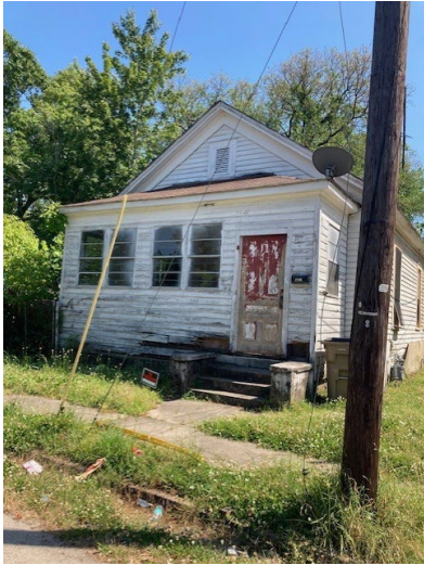
1. View of façade, looking SE
