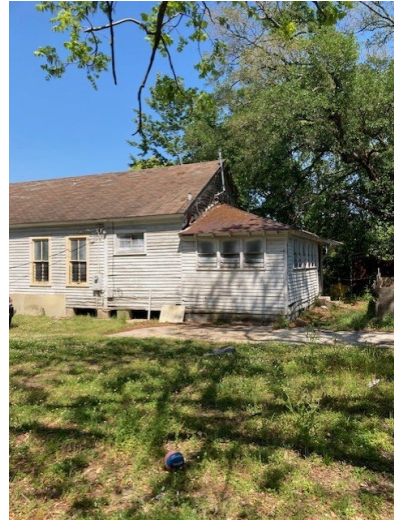
2. View of west elevation, looking E
