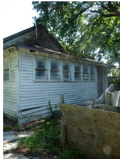
4. View of south elevation, looking NE.
