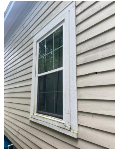
4. Detail of window on north elevation
