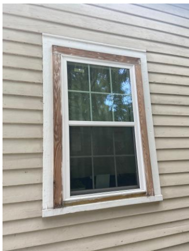
5. Detail of window on north elevation
