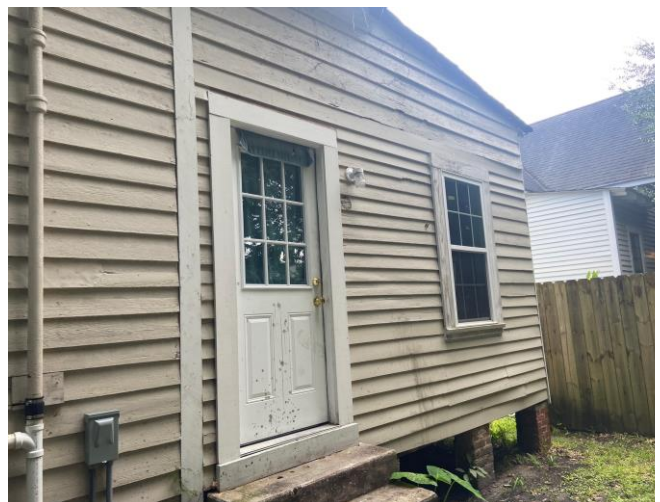
6. View of rear elevation, looking SE
