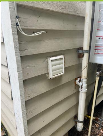
7. Detail of rear elevation
