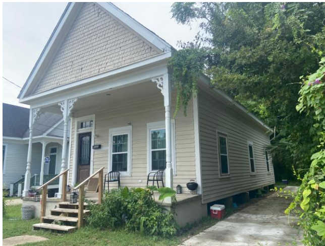
3. View of façade and north elevation, looking SW
