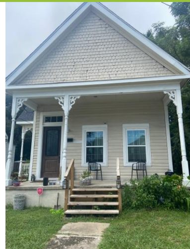
2. View of façade, looking W
