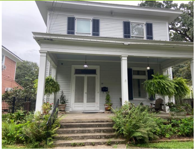
2. View of façade, looking E
