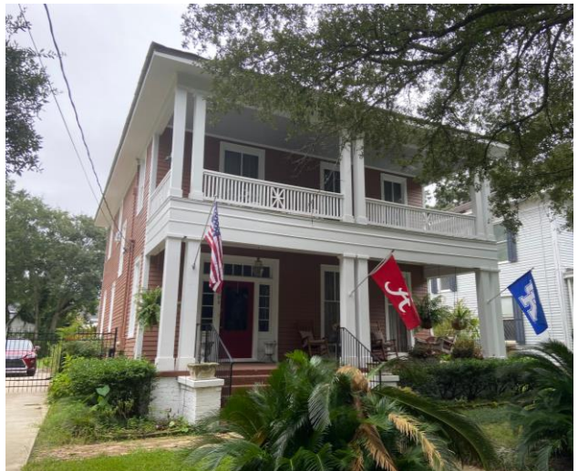
6. View of façade arrangement at adjacent property, 309 S Ann
