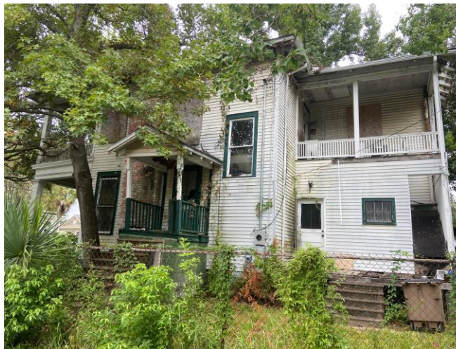
5. View of east elevation, looking W
