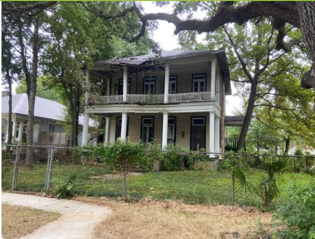
1. View of façade, looking S
