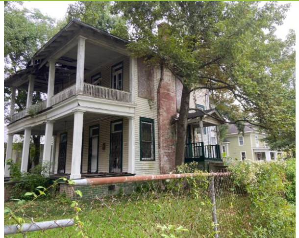
2. View of east elevation, looking NW
