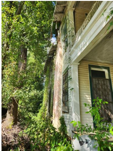
3. View of west wall, looking N
