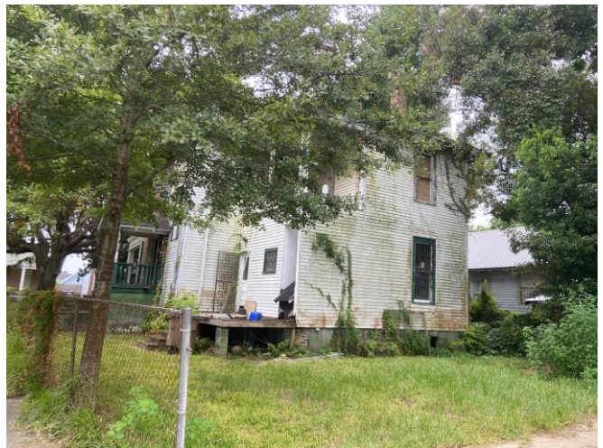
6. View of north (rear) elevation, looking SW
