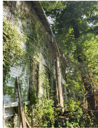
4. View of west wall, looking SE
