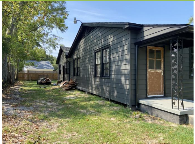
2. View of west east elevation, looking S
