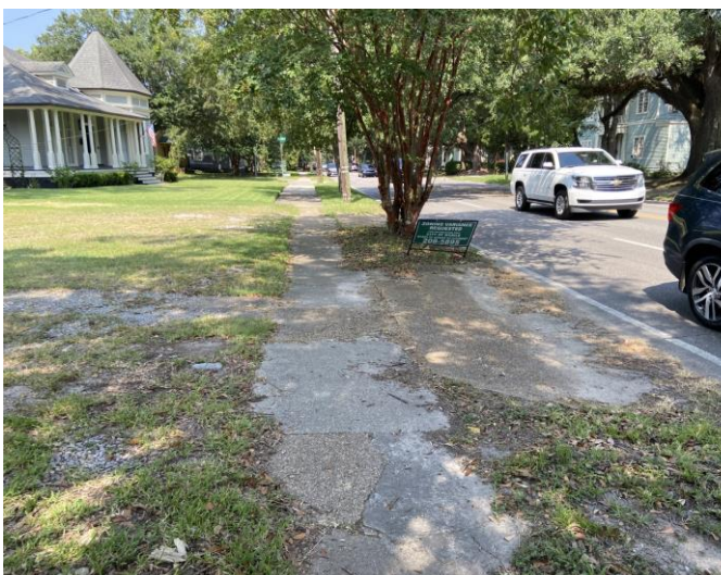
5. View of ROW and evidence of prior front paving
