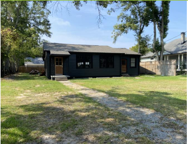
1. View of property looking SW
