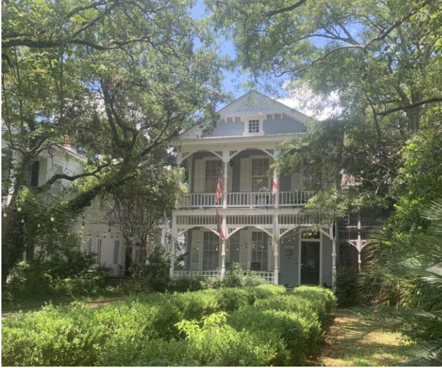
1. 962 Dauphin south façade, looking north.
