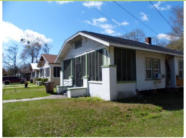
2. View of property, looking southwest
