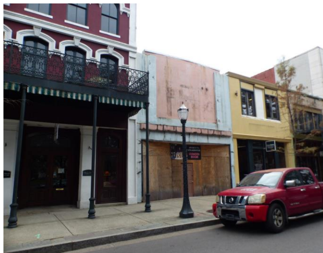
2. View of property, looking southwest
