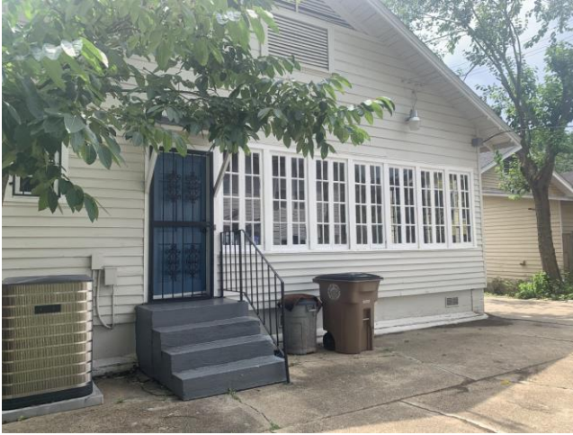
7. View of west (rear) elevation, looking southeast.
