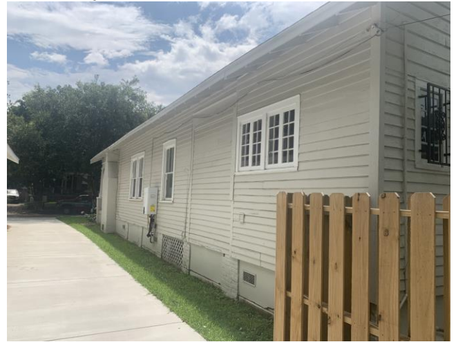
4. View of north elevation, looking southeast (note the evidence of a rear addition). All side elevation windows would be replaced with vinyl sashes.
