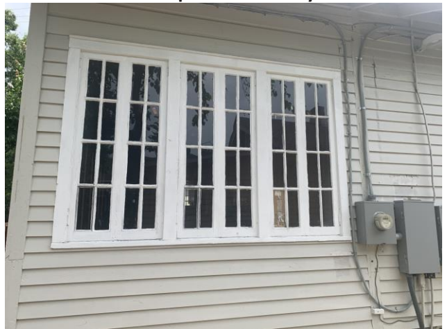
6. Detail of sunroom windows to be removed on south elevation.
