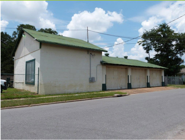
1. View of south façade, looking NE
