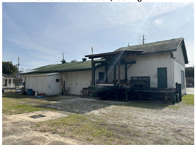
6. View of north (rear) elevation, looking SE
