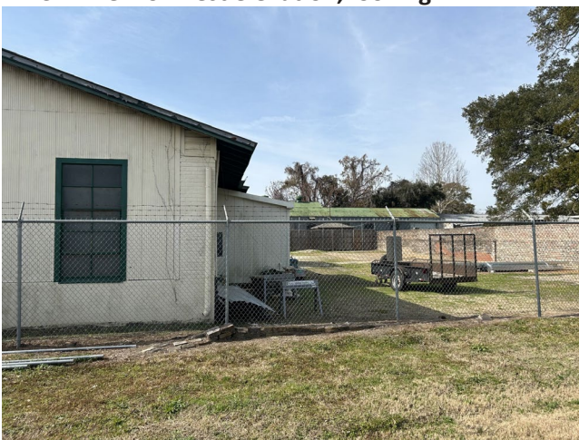
5. View of east elevation, looking W
