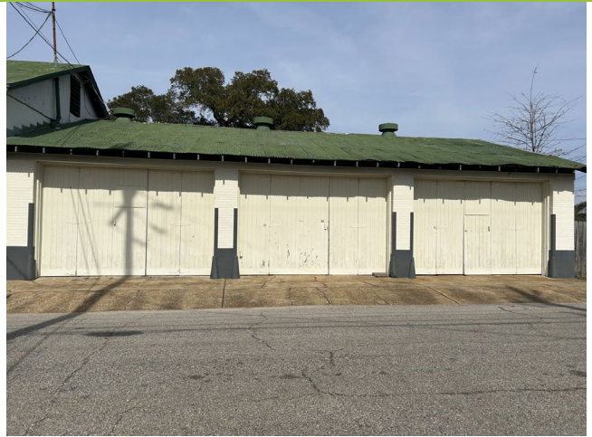
2. View of south façade, looking N
