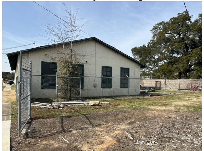
4. View of east elevation, looking NW
