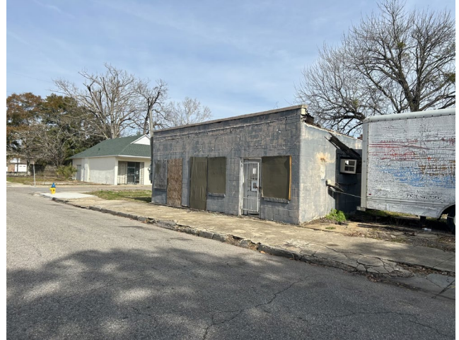
2. View of façade, looking NE
