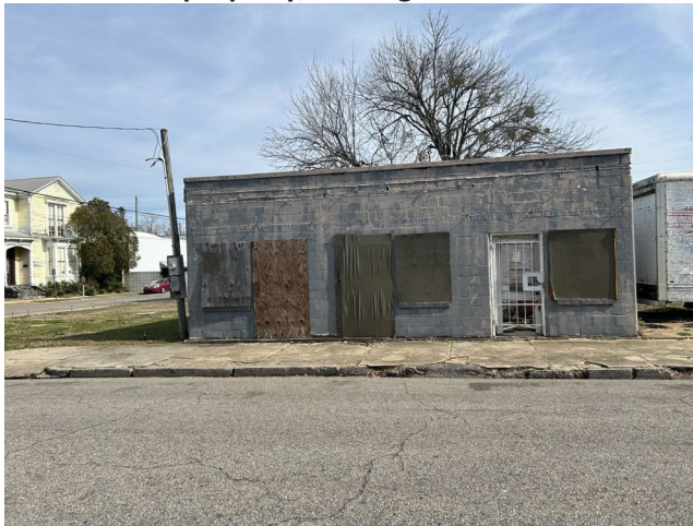
3. View of west façade, looking E
