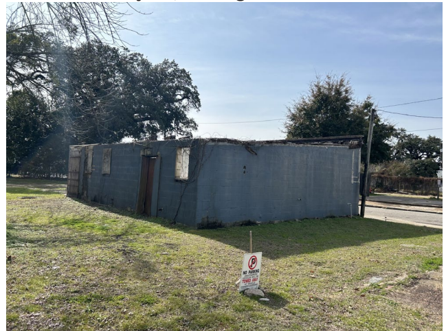
4. View of north and east elevations, looking SW
