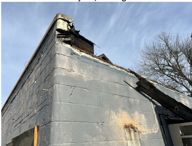
5. Detail of structure's condition
