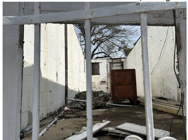
6. Detail of structure's condition
