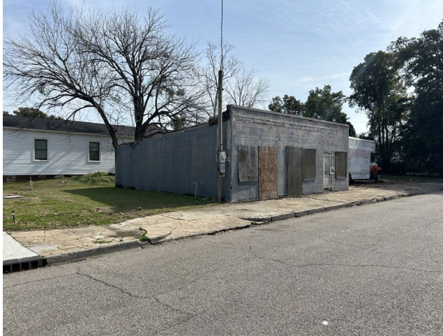
1. View of property, looking SE
