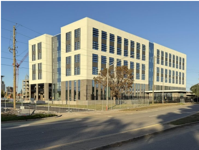
1. South façade, looking NE across Canal Street
