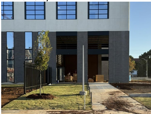
5. Entrance vestibule, looking S
