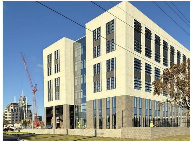
2. West elevation, looking NE from driveway entrance on Canal Street
