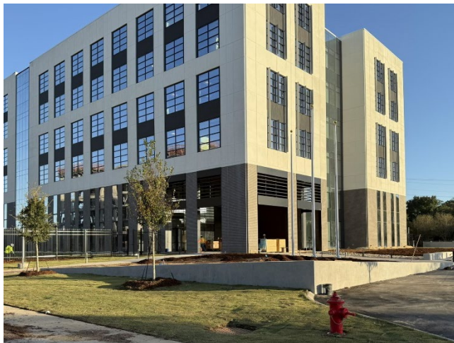
3. North and west elevations, looking SE from driveway
