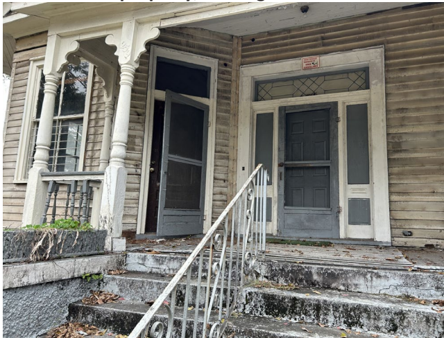
3. Detail of front porch and doors to be removed.
