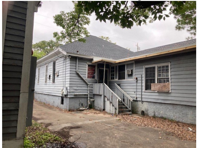
4. View of south elevation, looking NW
