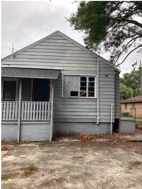
5. View of east (rear) elevation, looking W
