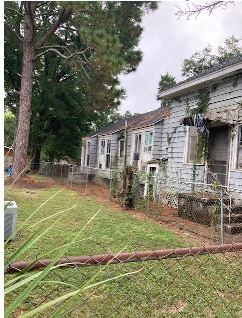
6. View of north elevation, looking E
