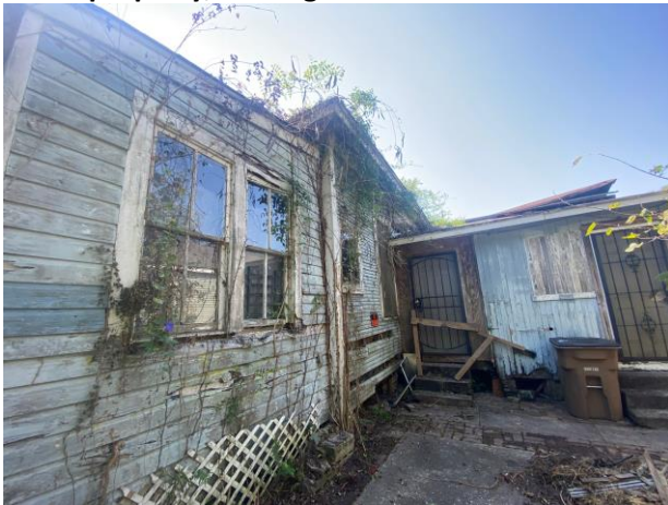
3. View of rear elevation with additions, looking W.
