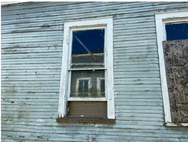
5. Detail of window on north elevation
