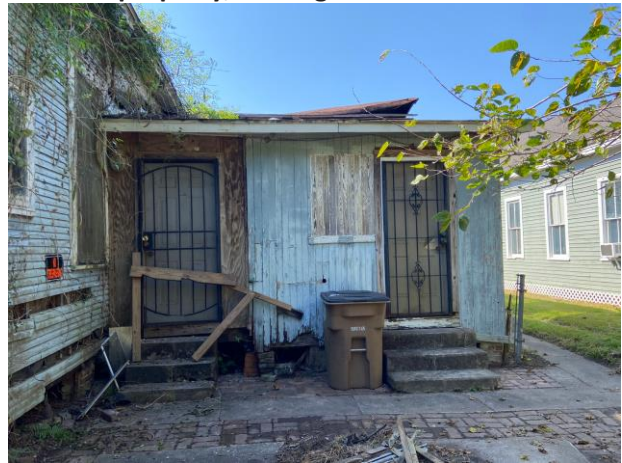
4. View of addition on north end of rear elevation, looking W
