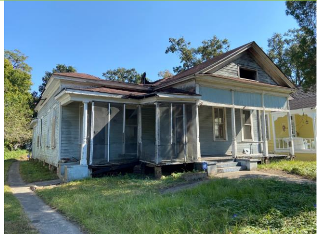
2. View of property, looking SW
