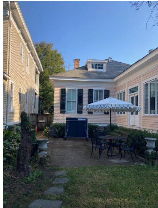
4. View of south elevation of main block, looking N
