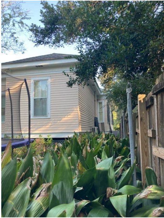
5. View of south and east elevations, looking NW
