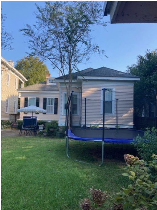
3. View of south elevation, looking N
